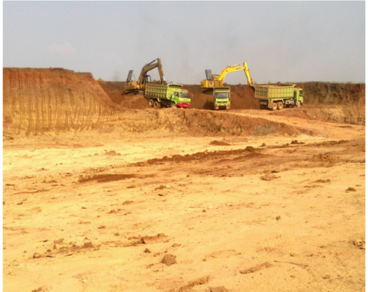
Cut and Fill Work in Phase 3
